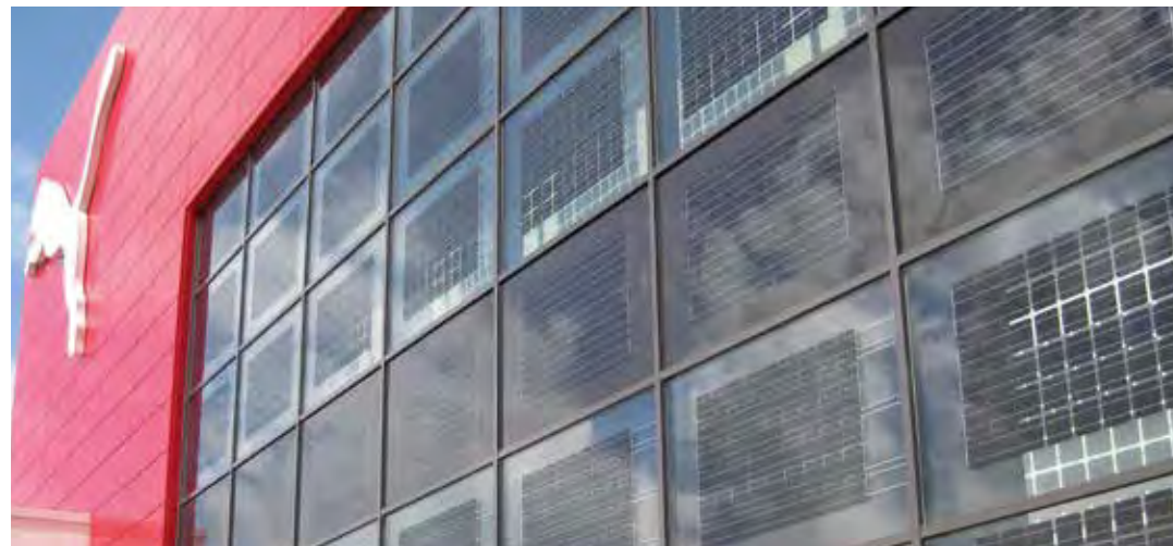
Generation and usage of solar power at PUMAVision Headquarters in Herzogenaurach
